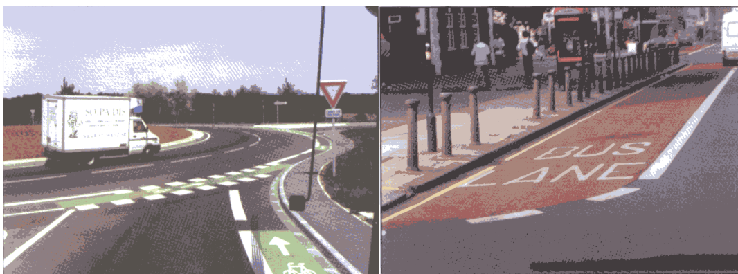
Green pavement where bike lane intersects vehicle lane, France.
