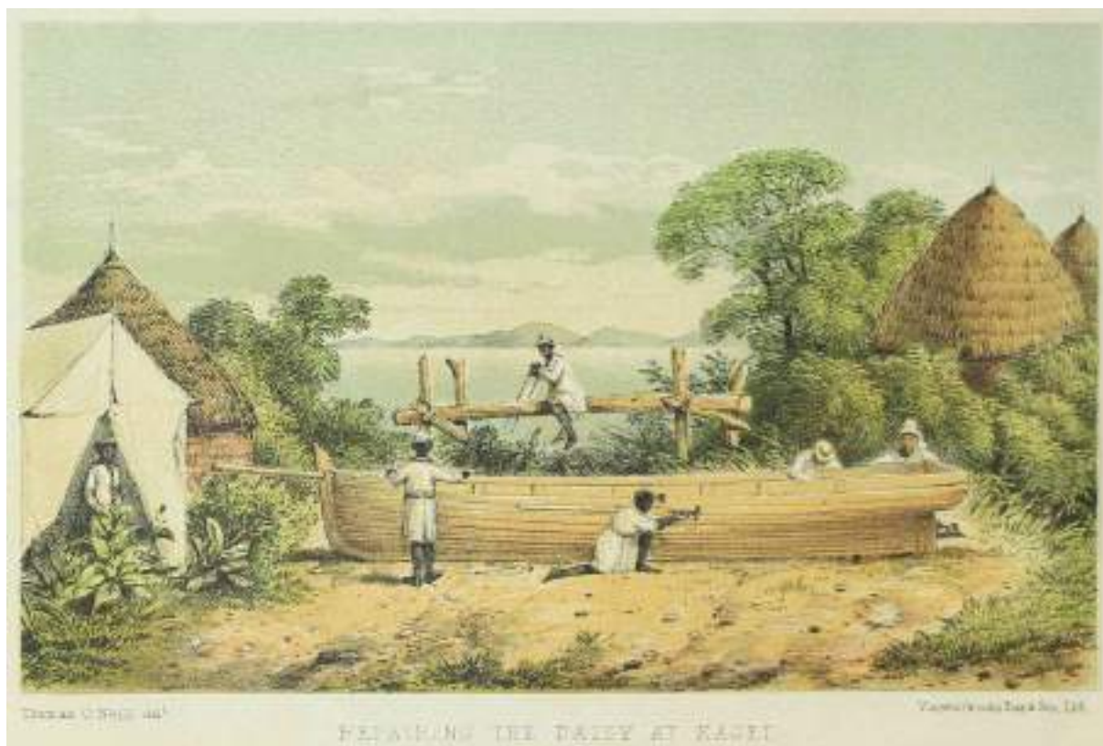
Figura 8 - Repairing the Daisy at Kagei
