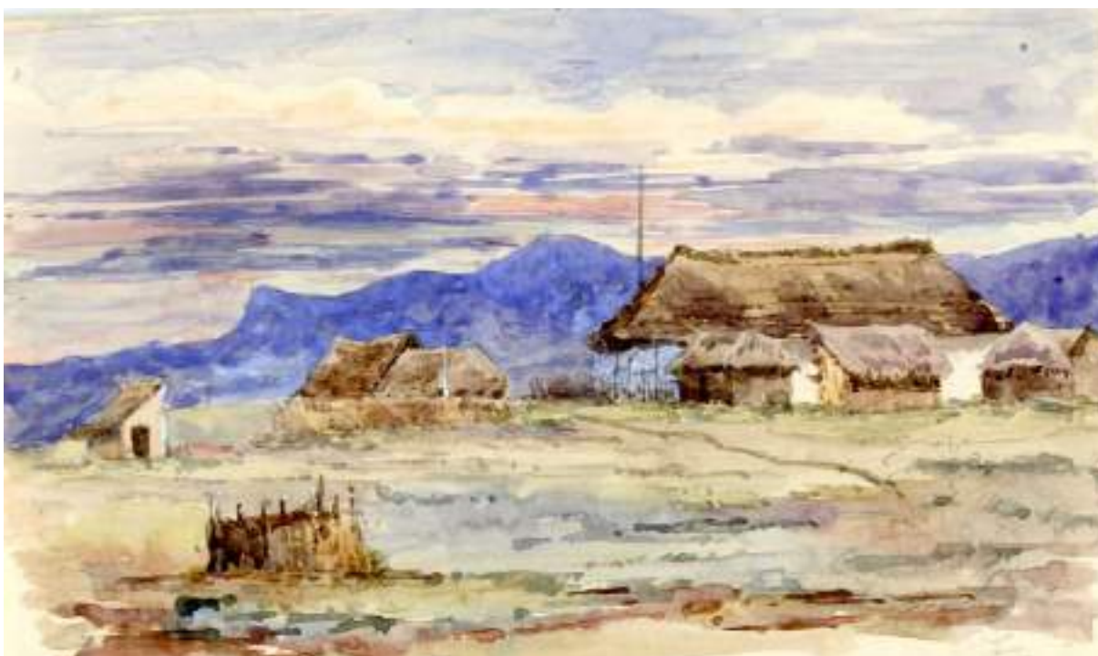
Figura 5 - Telegraph Station, Uganda Railway
