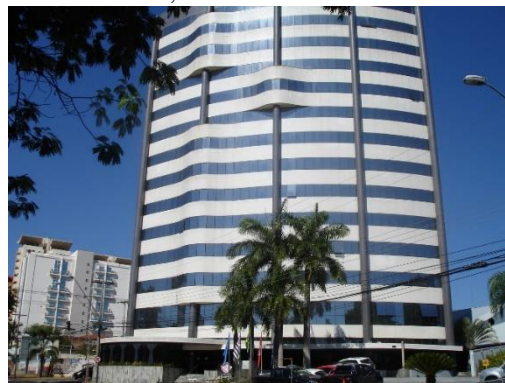
Figura 74. Fachada do Quality Hotel Saint Paul, na Avenida José Munia.
