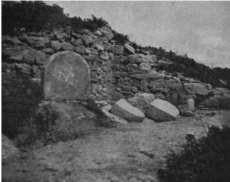
Figure 34 - Semi-circular limestone merlons of the battlement
