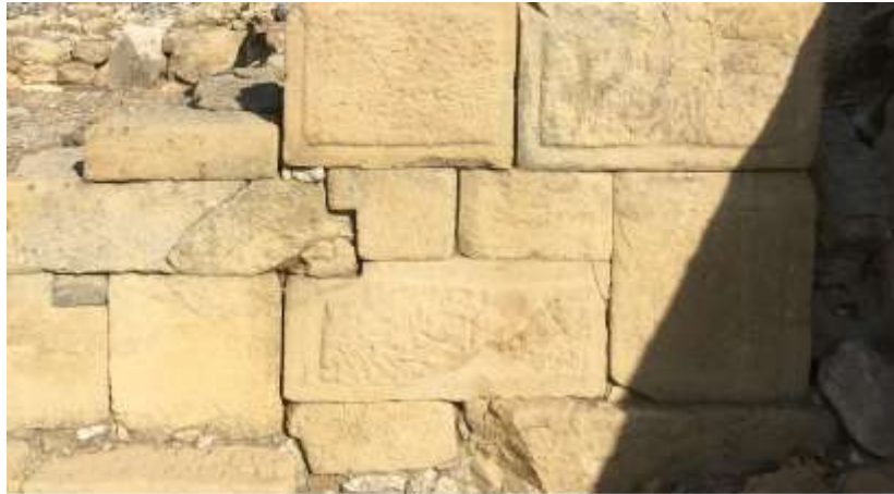
Figure 103 - Example of bossage in ashlar at Carteia and two other similar styles
