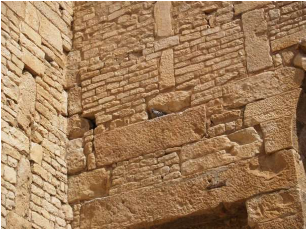
Figure 61 - An example of opus africanum wall in Dougga (Tunisia)
