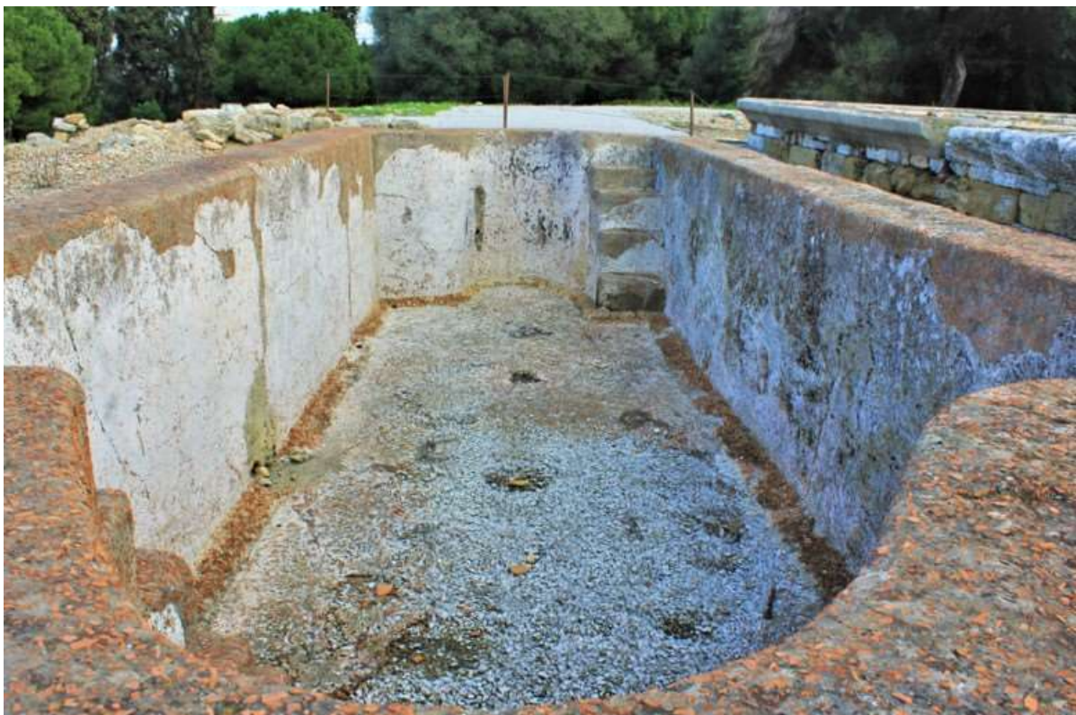
Figure 117 - Image of the sacred pool, showing the use of hydraulic mortar similar to that used in the staircase of the Roman temple.
