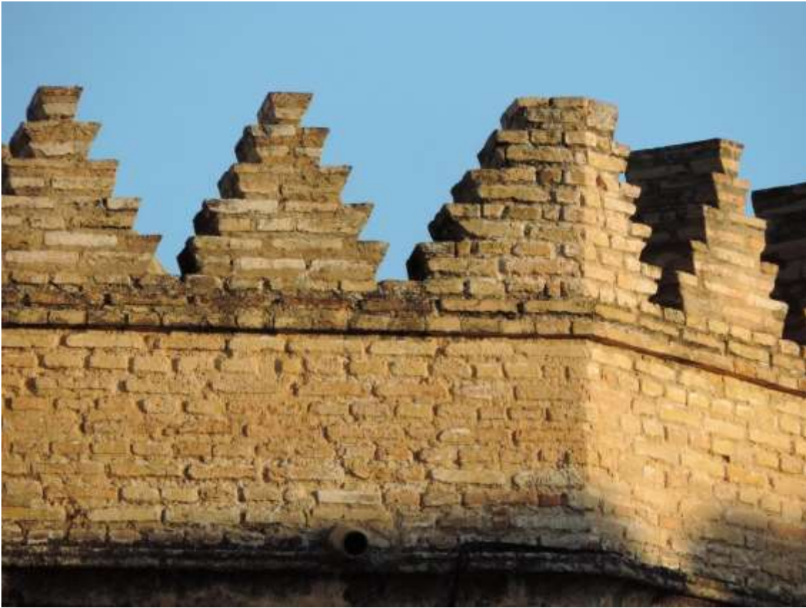
Figure 12 - Example of triangular merlons in Seville from the Islamic period
