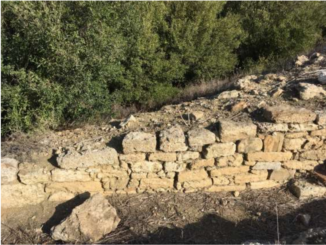
Figure 109 – View of Tramo 3
