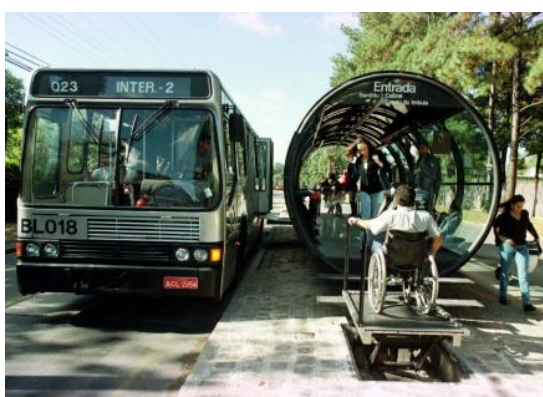
Figure 18 – Tube station belonging to RIT, Curitiba’s BRT system. These stations allow accessibility for people with disabilities and fare prepayment.
