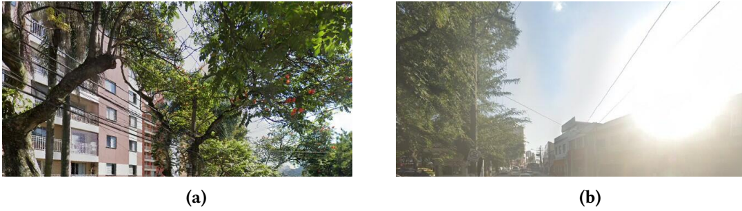
Figure 6.1: Images from Google Street View. (a) Trees are in contact with electrical wires. (b) Bad visibility due to sun glare.
