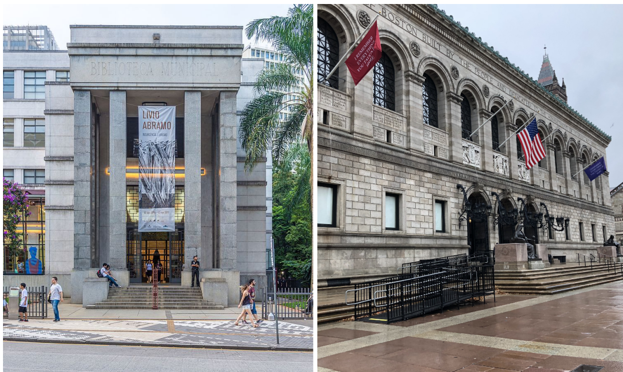
Figure 3.1: Historical lack of accessibility: on the left: Mário de Andrade Library (1940s) in São Paulo, Brazil. Handrails at the central section of the stairs and tactile flooring on the sidewalk pavement are modern additions for improving accessibility. On the right: McKim Building of the Boston Public Library (1895) in Boston, United States. Metallic ramps were installed to allow wheelchair users to enter the building. In both cases, later architectural interventions are intentionally designed to be visually distinct from the buildings to preserve their original appearance. Image sources: (Wikipedia, 2021a) (left) and Author (right).
