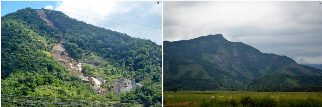
Figure 5 – Santo Antônio Hill, Caraguatatuba (a) Landslides in 2017 and (b) Landslide scars
