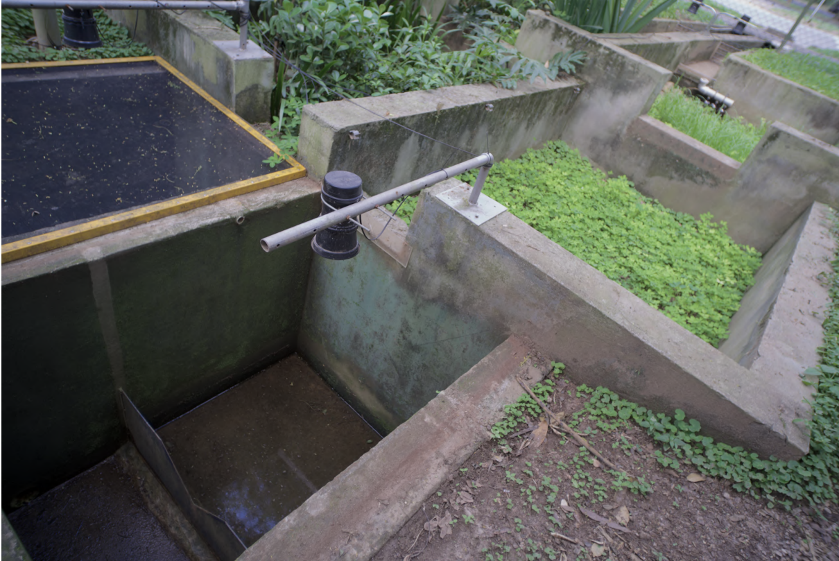
Figure 27 – Bioretention using the same method for water quantity characterization: inlet with a rectangular-notch acrylic thin plate weir surrounded by a concrete framing and outlet with a triangular-notch steel thin plate weir in a concrete tank.
