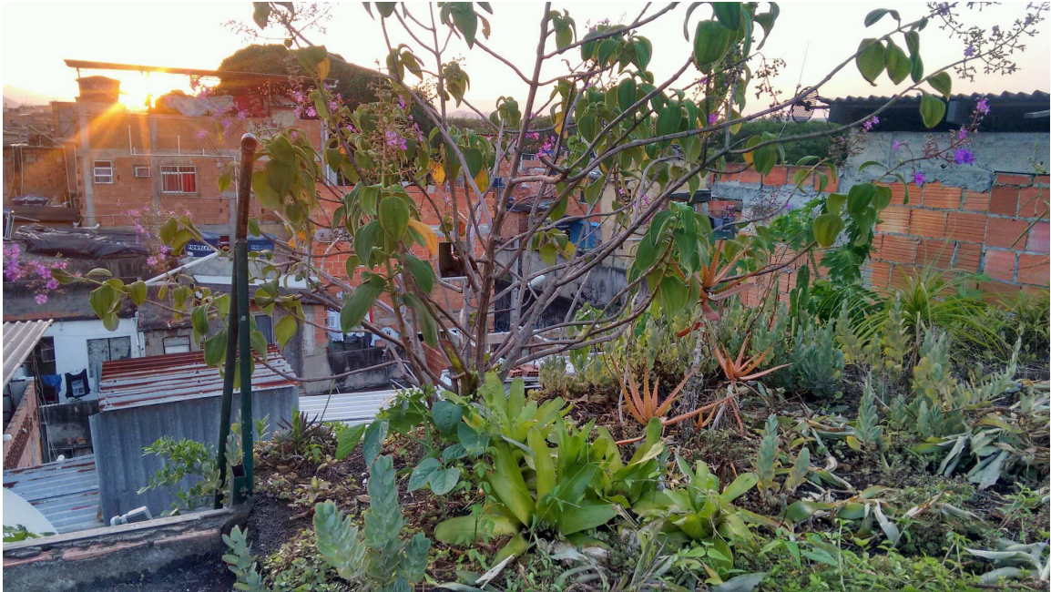
Figure 48 – Vegetated roof installed in the community of Parque do Arará in Rio de Janeiro, in the northern zone city slums, part of the “Teto verde favela” project.
