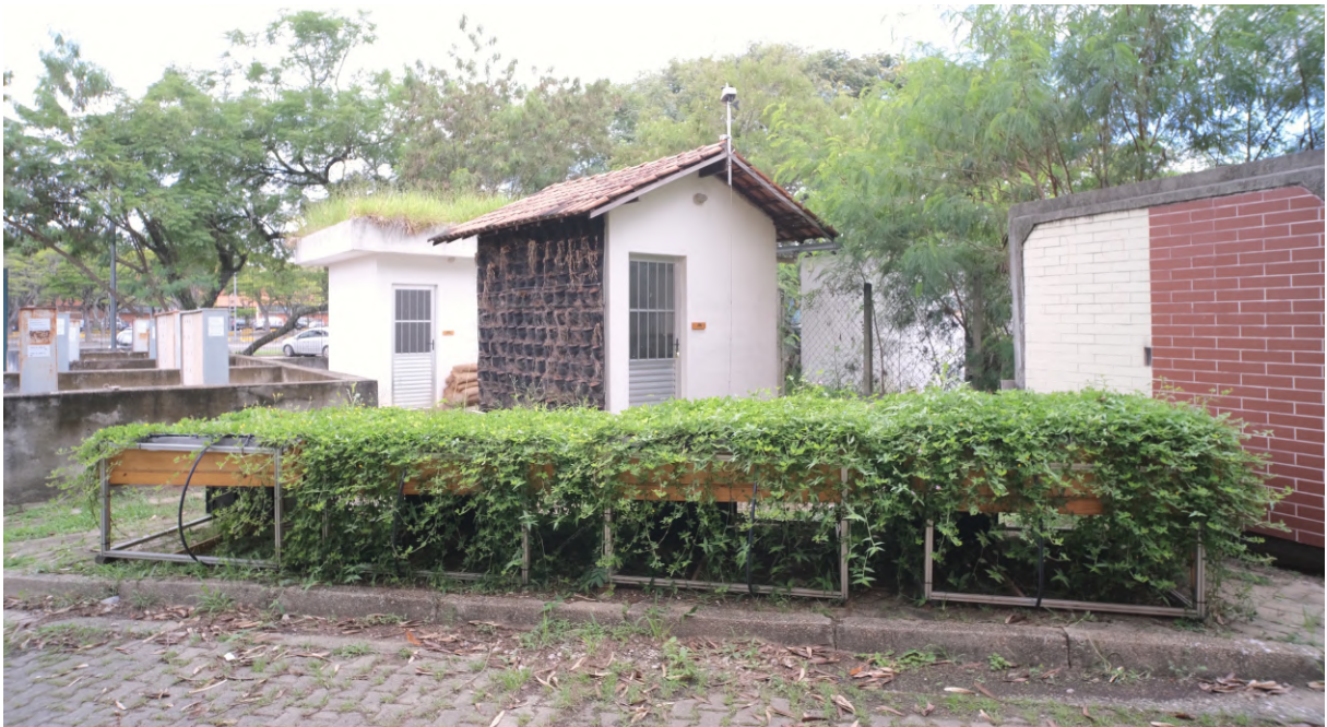
Figure 31 – Experimental setup. Buildings on the back are the unmanaged vegetated roof (VR) and the ceramic tiled (CT) masonry prototypes. Testbeds on front are the unmanaged M1, M2, M3 and M4 models from right to left, with respectively 200 mm, 150 mm, 100 mm and 60 mm substrate depth.
