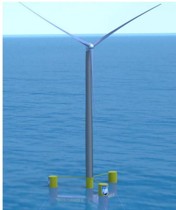
Figure 2.6: The UMaine VoltornUS-S reference platform designed to support the NREL IEA-15 MW system definition [45].
