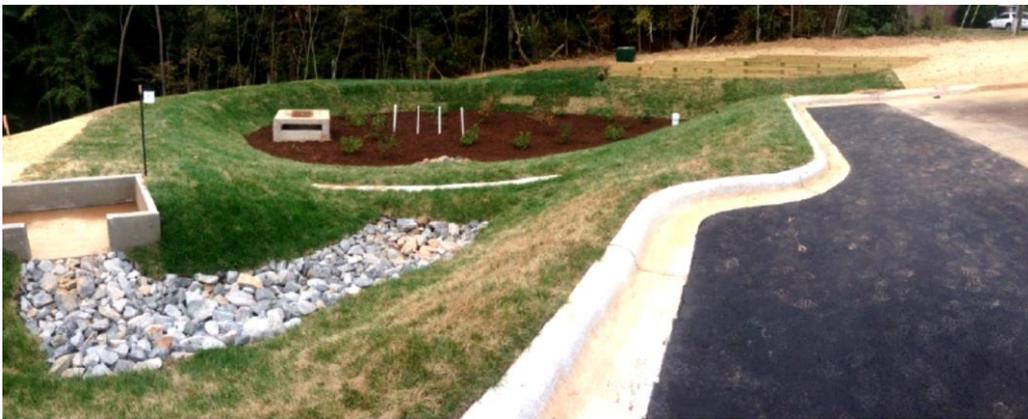
Figure 21 - Bioretention Area
