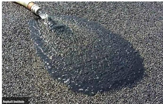
Figure 28 - Porous asphalt
