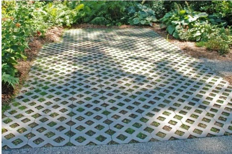
Figure 26 - Permeable paver
