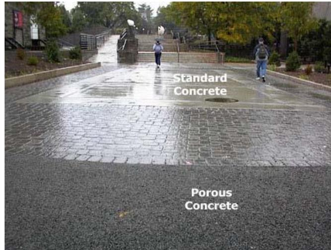
Figure 27 - Porous concrete
