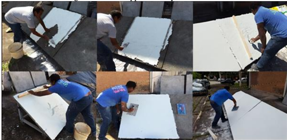
Figure 5. Mortar application by mason in situ
