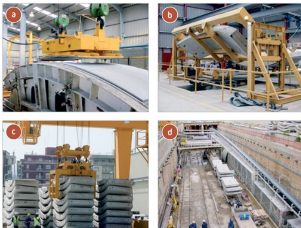
Figure 1-Transitional loads in construction stages of a TBM tunnel: (a) demolding, (b) handling, (c) stocking, and (d) transportation. (de la Fuente, 2017)
