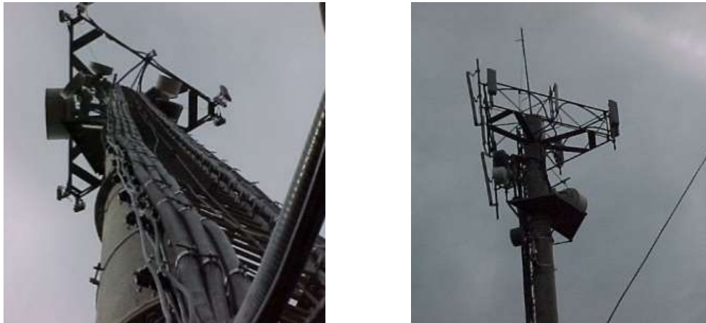
Figure 2 - Pictures of the reinforced concrete pole
