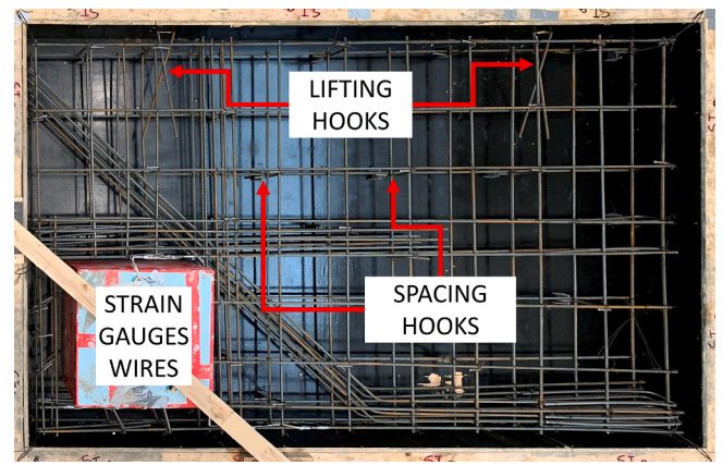
Fig. 12. SI.a formwork before the casting.
