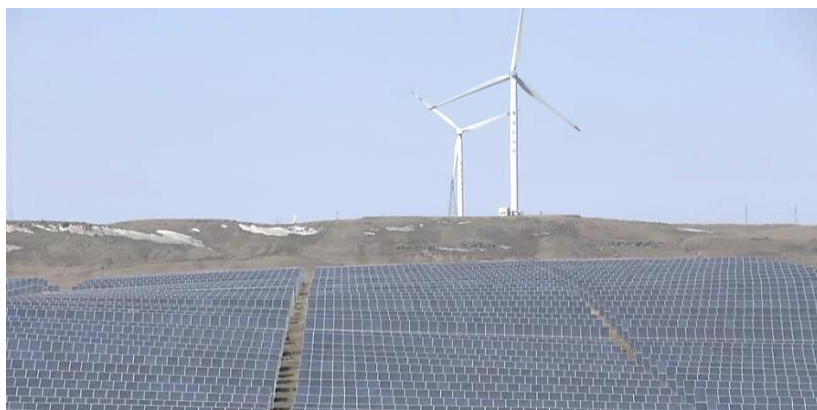
Figura 19 — Luneng Haixi Multi-Mixed Energy Demonstration Project, Golmud
