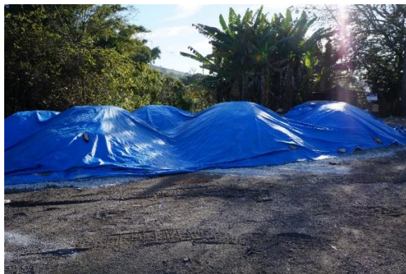
Figure 41 - Stockpiles covered with impervious blanket
