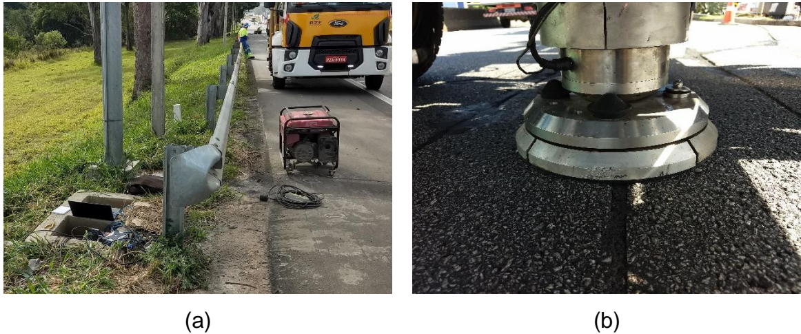
Figure 62 - Setup for field measurement and FWD test being carried out
