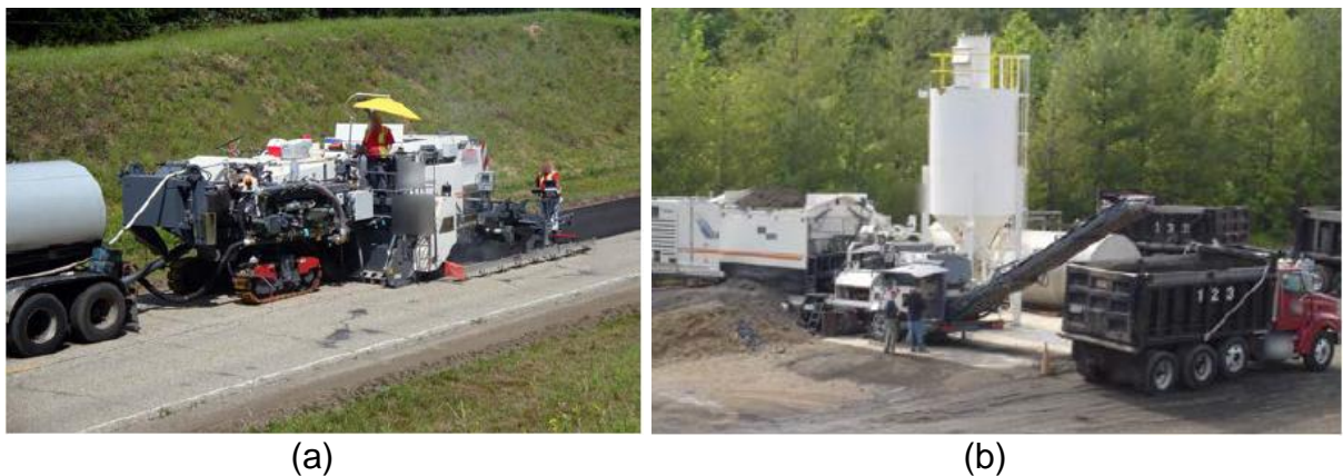
Figure 3 - Examples of (a) CIR and (b) CCPR process
