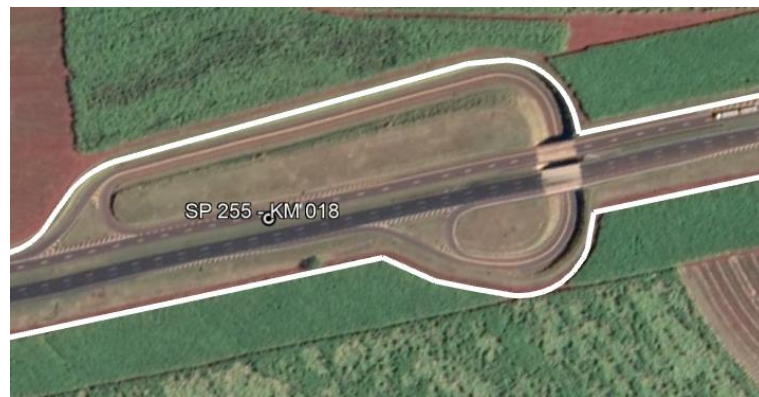
Figure 13 - U-turn highway ramps overpass bridge
