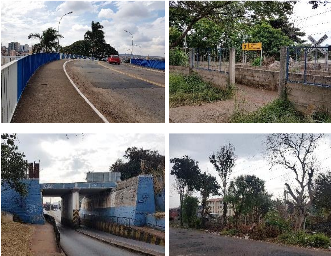
Figure 4.4 - Examples of types of crossings and segments without railroad crossings. From top left to bottom right: OP1, PC2, UP4 and SWC6
