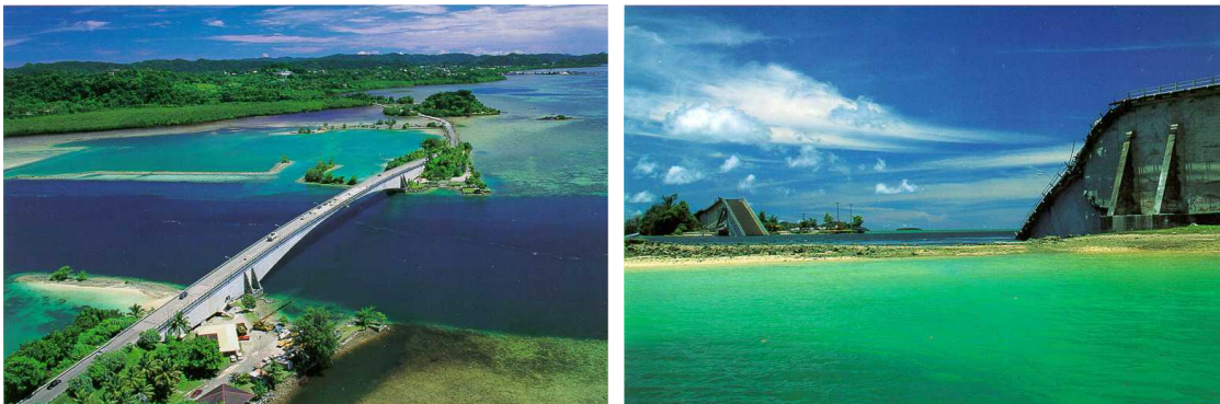
(a) Ponte Koror-Babeldaob
