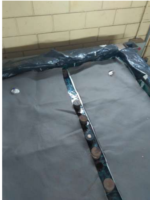
Figure 5.21: Non-woven geotextile sheets placed over airbags to minimize friction with plywood boards.
