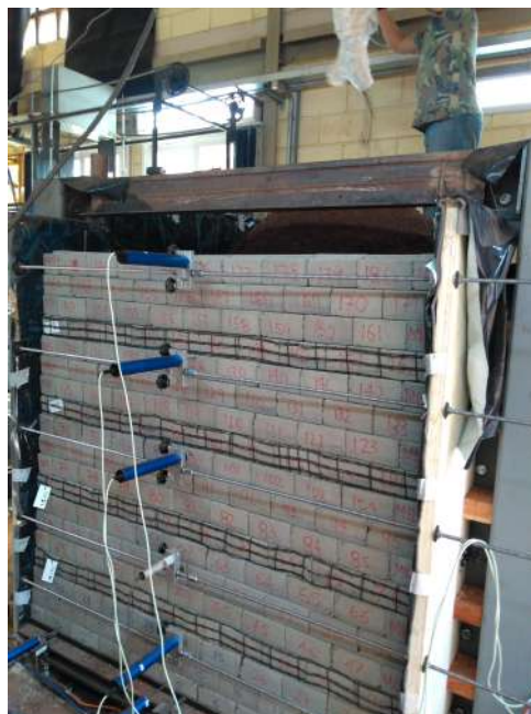
Figure 5.18: Transversal rods mounted between the lateral plywood sheets to provide block lateral restraint and support for the facing displacement transducers during wall construction.
