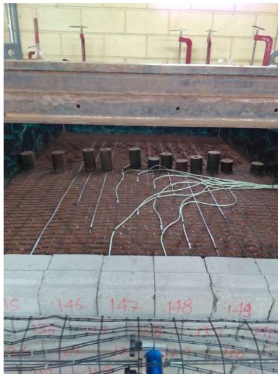
Figure 5.42: Extensometer wiring enclosed by plastic tubes, extended up to the rear wall.
