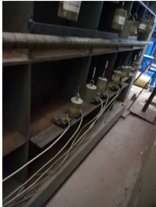
Figure 5.74: Manual extensometers connected to dead weights and draw-wire potentiometers (below) at the outside of the rear wall.
