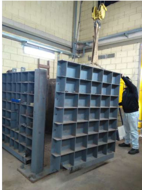
Figure 5.11: Removal of the front wall of the test box.
