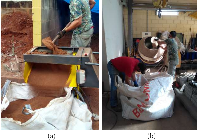
Figure 5.65: Soil preparation: (a) Soil sieving close to the outdoor soil stockpile; (b) Soil mixing and moisture adjustment.
