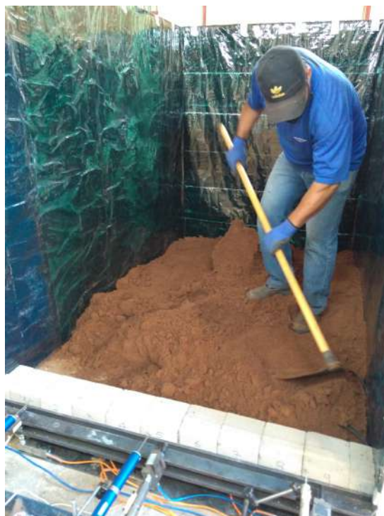
Figure 5.68: Soil spreading before compaction.
