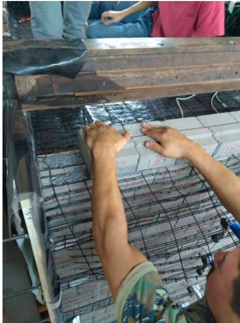
Figure 5.63: Block placement at the wall facing.
