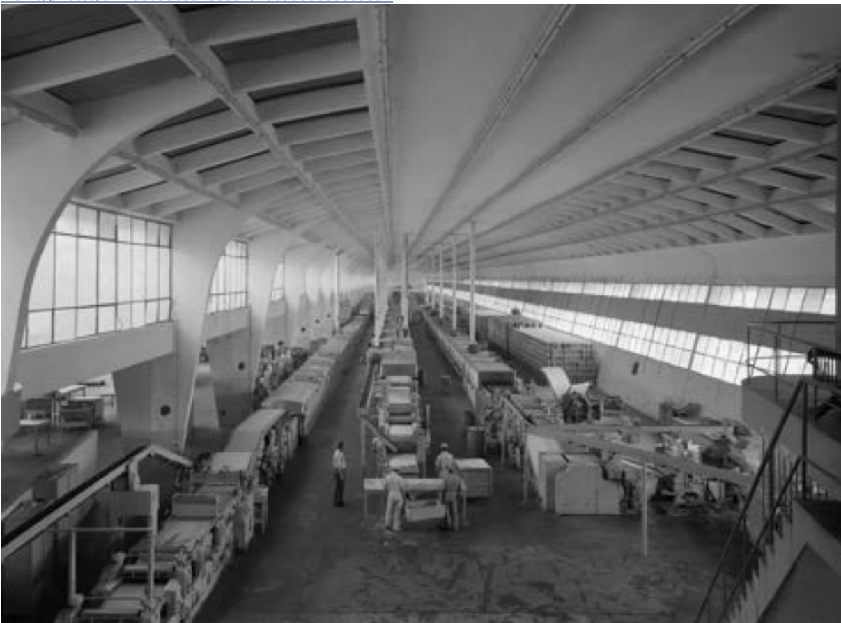
Figura 4-92 – Vista interna da fábrica – Hans Gunter Flieg © IMS Fote: https://www.facebook.com/oscarniemeyer-works/photos/a.1408658639403597/2069300603339394
