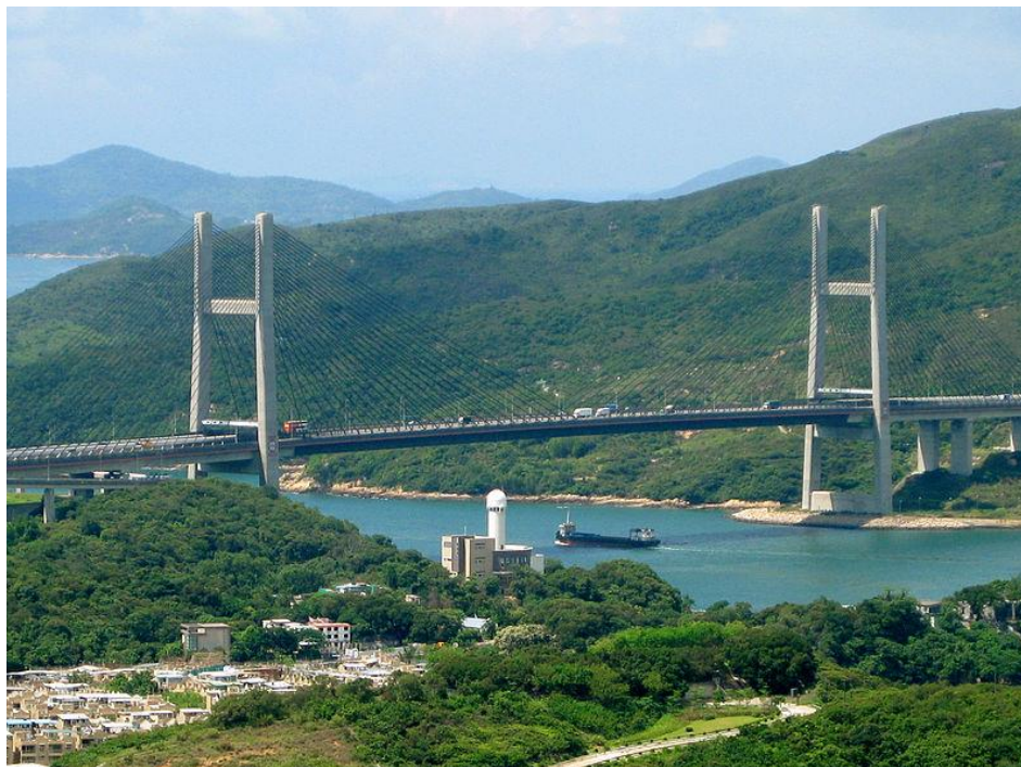
Figura 69 - Ponte Kap Shui Mun, Hong Kong.
