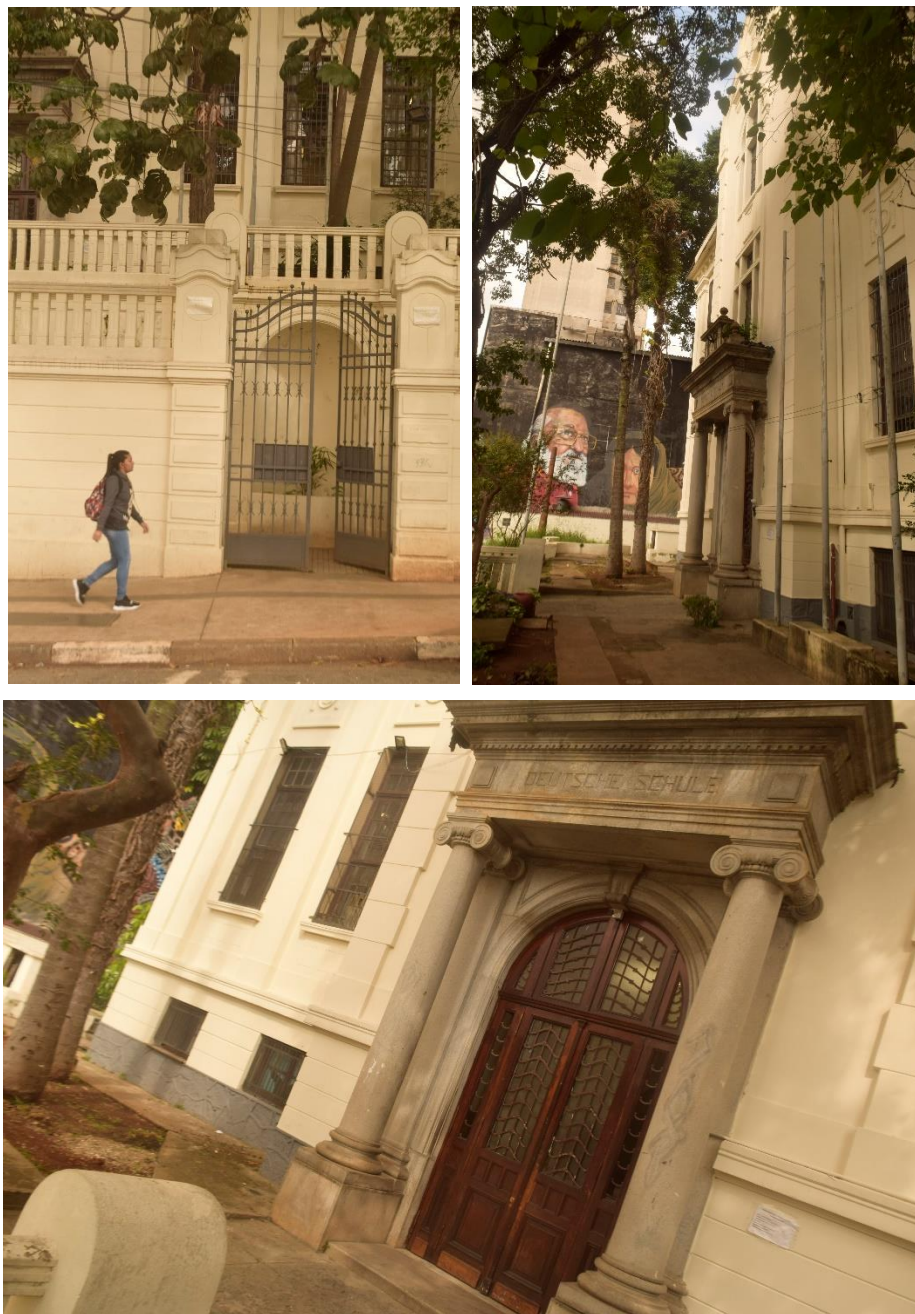
Figura 41: ECS A – Walk-around-the-blocks - entrada
