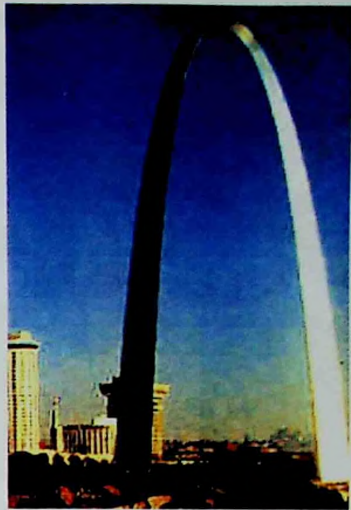
Figura 129: Gateway Arch of Saint Louis
