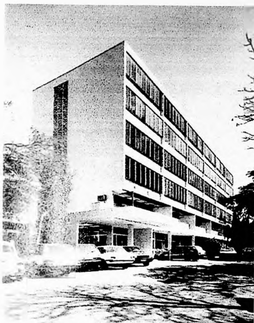
Hospital Infantil do Morumbi, 1951 Hospital de Vila Serra do Navio, 1955 AACD, 1958
