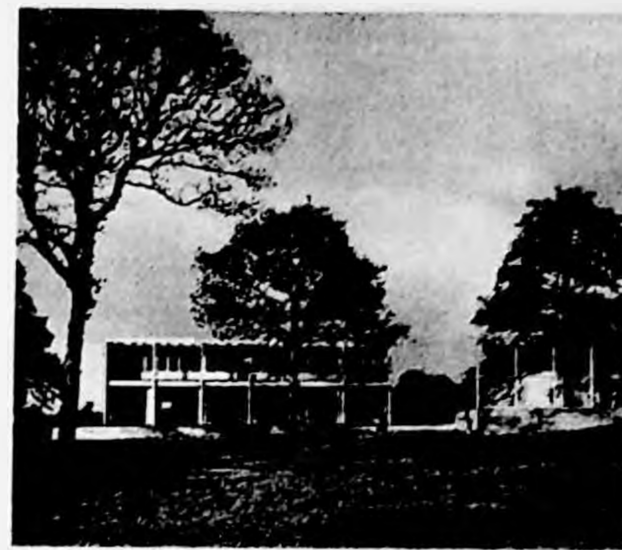
Christopher Tunnard (paisagismo) e Serge Chermayeff (arquitetura) Bentley Wood (Halland, Sussex), 1935 [TREIB, Modern landscape architecture , p. 147]
