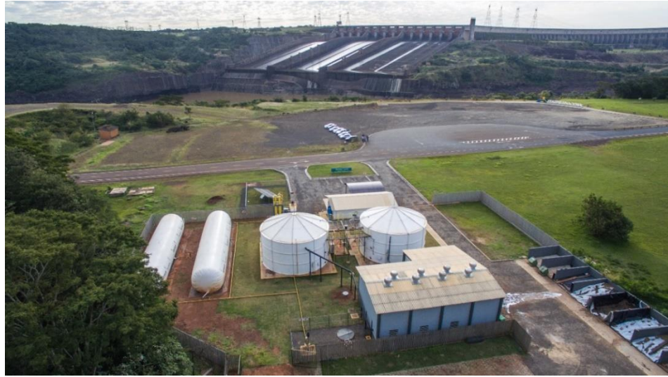
Figure 20: Waste treatment plant in Foz do Iguaçu, Brazil. Source: CIBiogas files.
