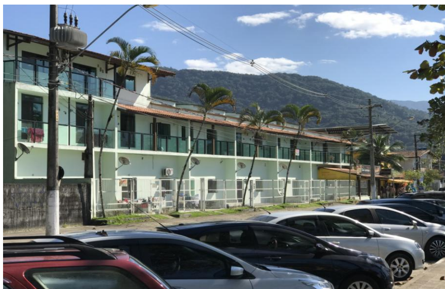
Figura 23 – Condomínio Residencial no Hotel Jangadeiro, 2019
