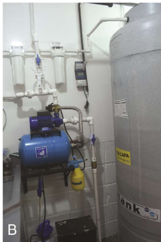
Fig. 7. A. Washing area and B. Filtering, storage and distribution water system of Laboratory of Experimental and Comparative Pathology (LAPECOM), School of Biology. University of Costa Rica. This laboratory was designed and built based on the project that represents these thesis.
