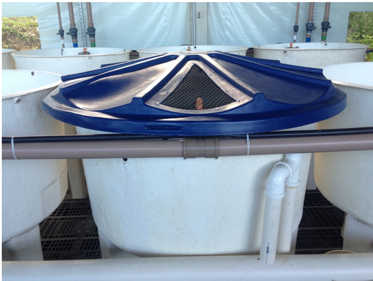
Figure 7 The plumbing supply consisted of PVC pipes with different diameters for income and effluent water.
