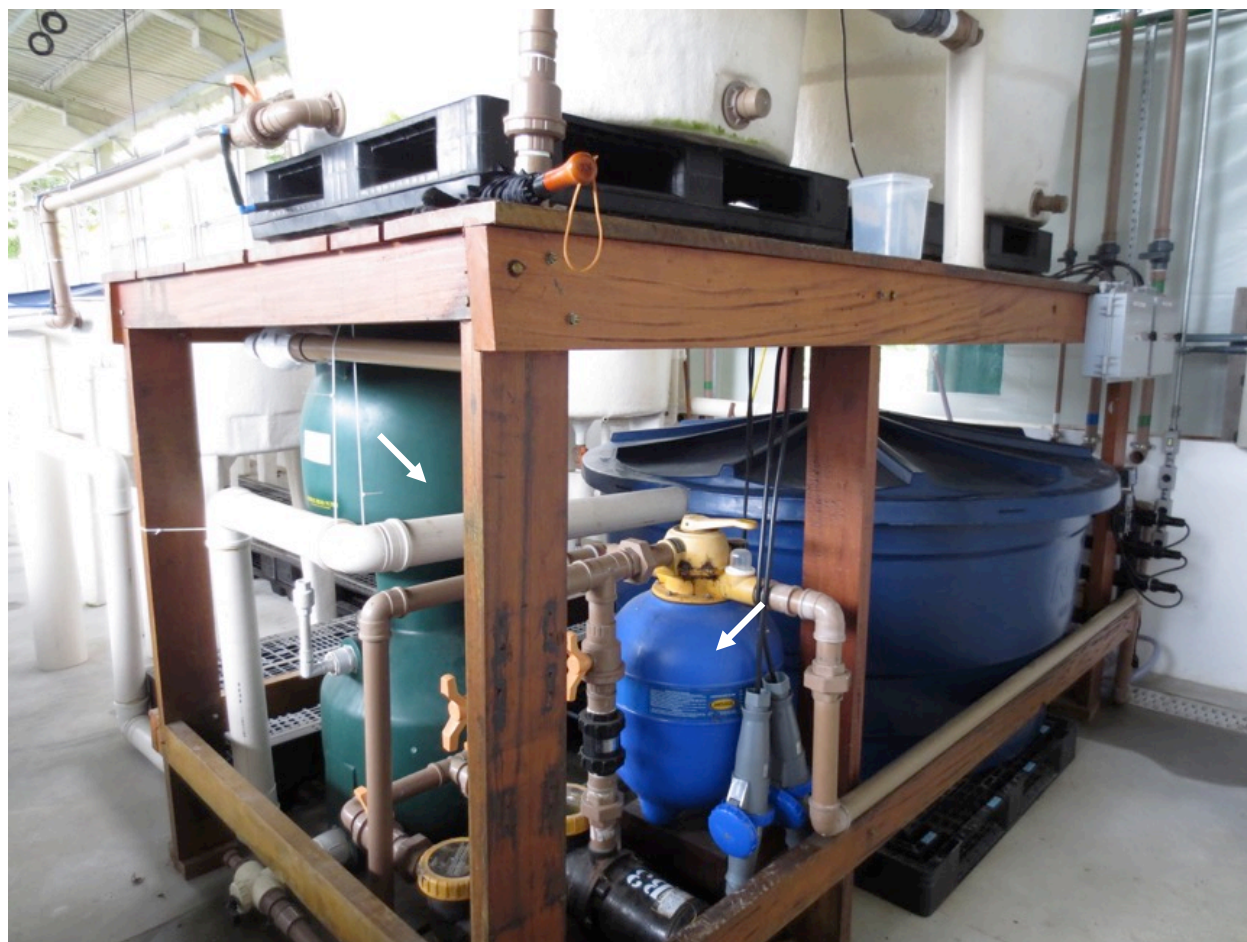
Figure 8 Water filtration system: sand filter (blue, right white arrow) and the bead filter (green, left white arrow), which performs the mechanical and biological filtration, respectively.
