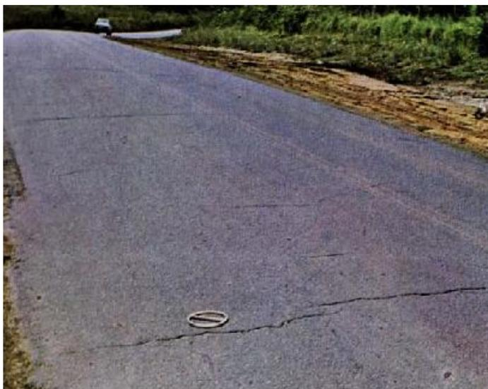
Figura 6 - Trinca transversal
