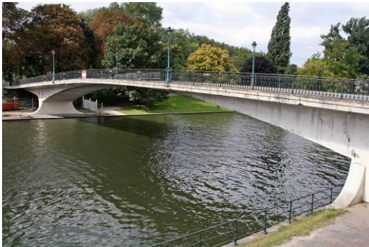
Figura 1. Mativa Footbridge. Liège. 1905.
