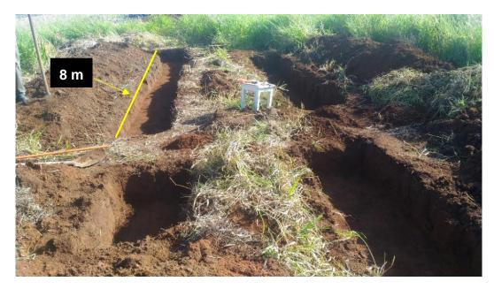
Fig. 3.4 Excavation of the ditches
