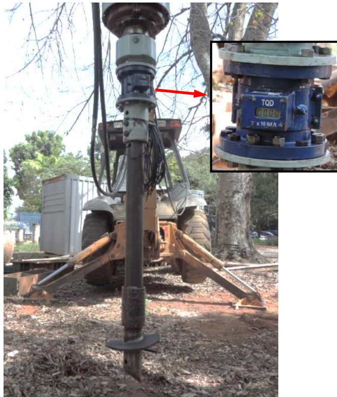
Figure 43. Installation of an instrumented helical anchor at the test site.
